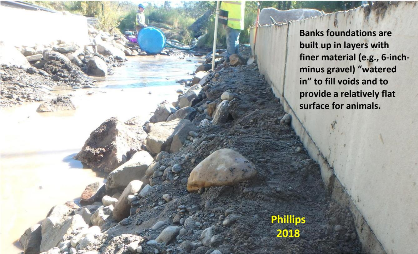
Banks foundations are built up in layers with finer material (e.g., 6-inch-minus gravel) “watered in” to fill voids and to provide a relatively flat surface for animals.
