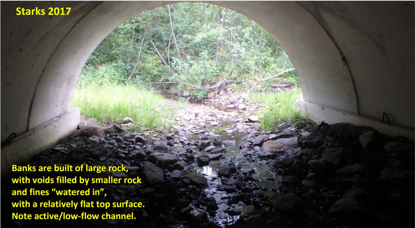
Banks are built of large rock, with voids filled by smaller rock and fines "watered in", with a relatively flat top surface. Note active/low-flow channel.
