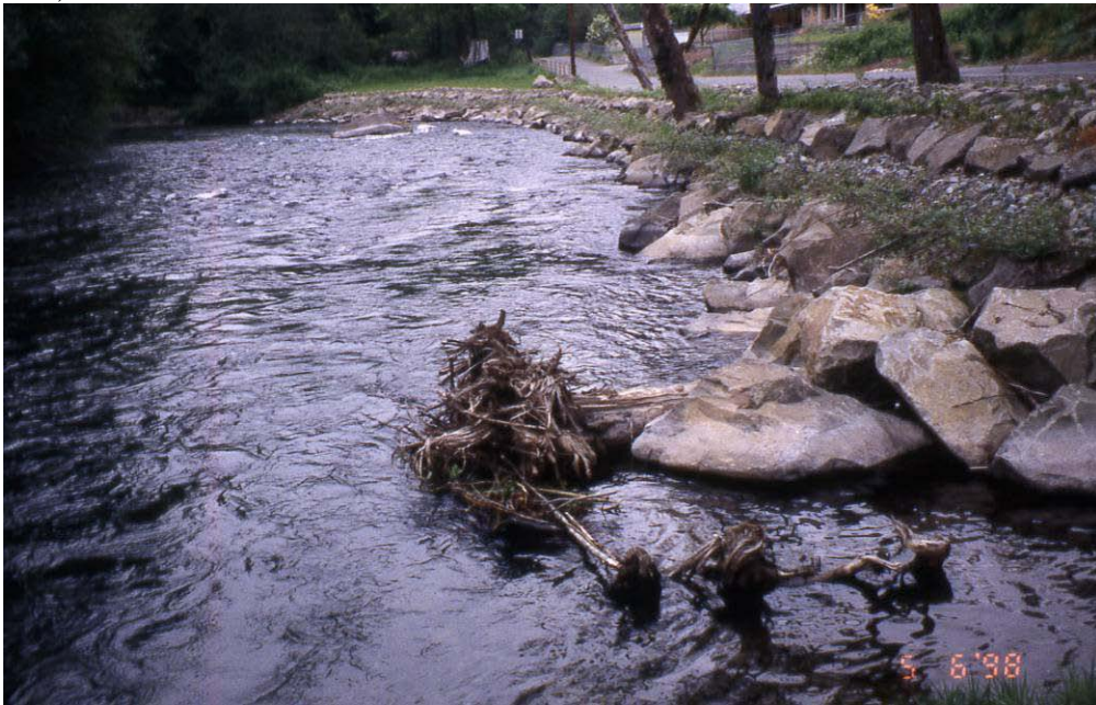
Figure 8. Large wood anchored in groin (Cedar River, Darre Dam project, King Co., WA).
