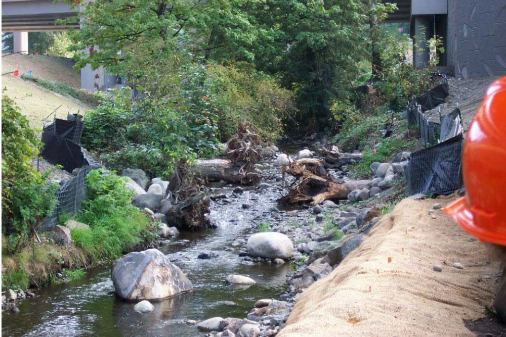
Figure 7. Habitat logs anchored in bank with additional boulder ballast (E. F. Issaquah Ck, I-90 Sunset Interchange, King Co., WA).
