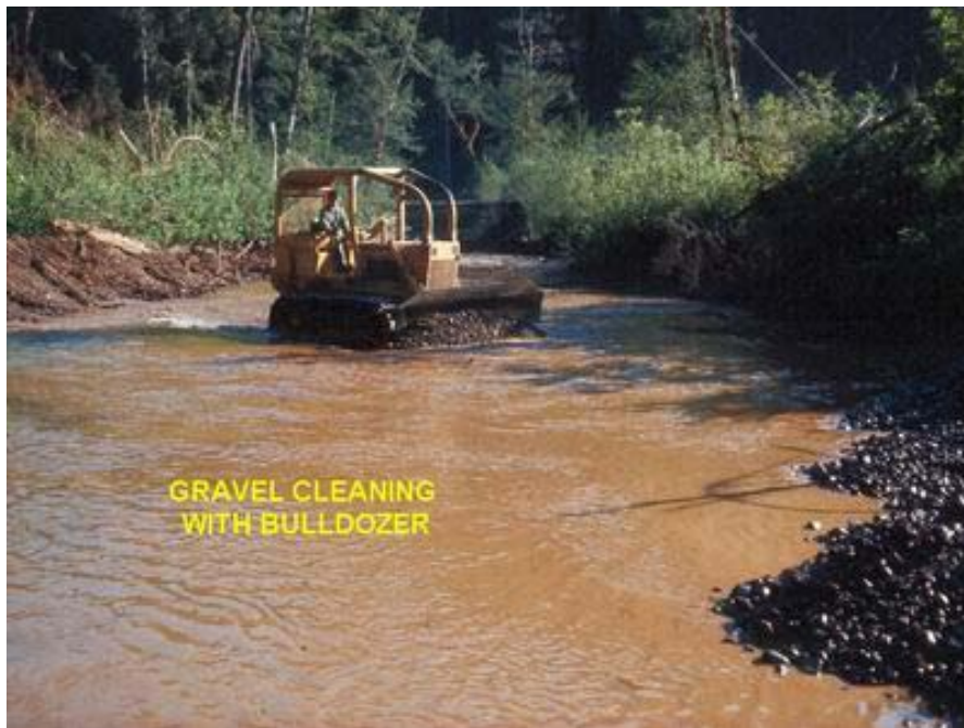
Salmonid Spawning Gravel Cleaning and Placement Figure 3. Gravel cleaning with bulldozer.
