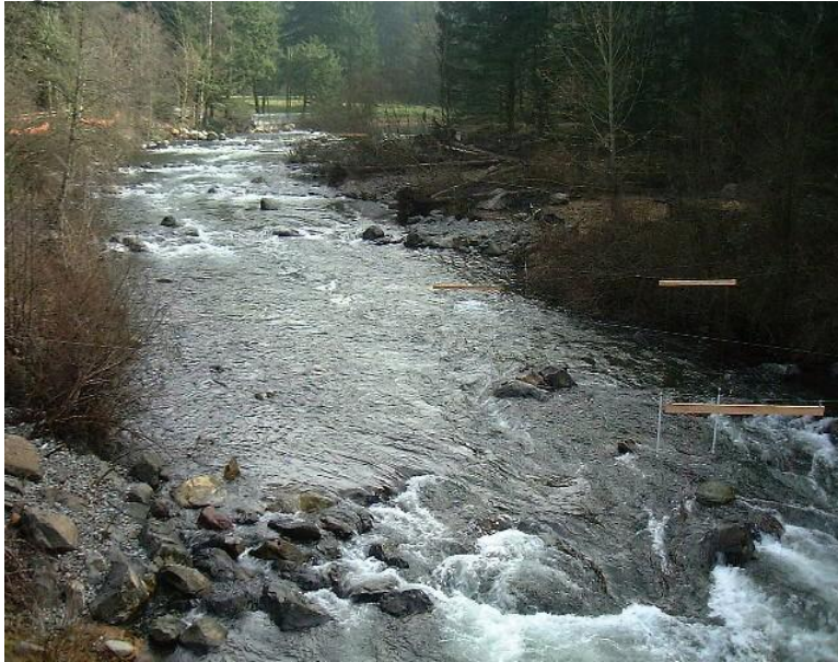
Figure 4. Porous boulder weir. Cedar River, WA.
