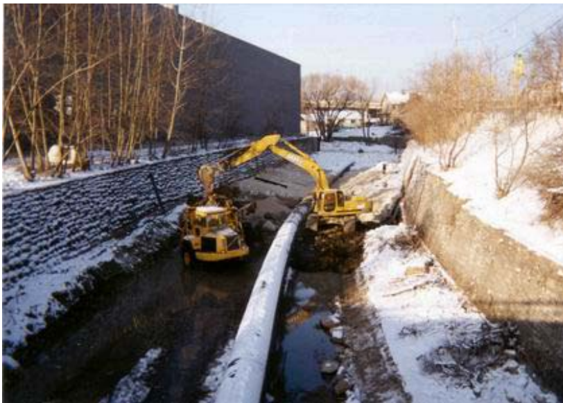
Figure 6. Dewatering an urban stormwater channel in preparation for stream restoration. The Menomenee River is diverted through a pipe, with coffers at each end defining the work area. Note track hoe on temporary in-channel pad. Source: Inter-Fluve, Inc.
