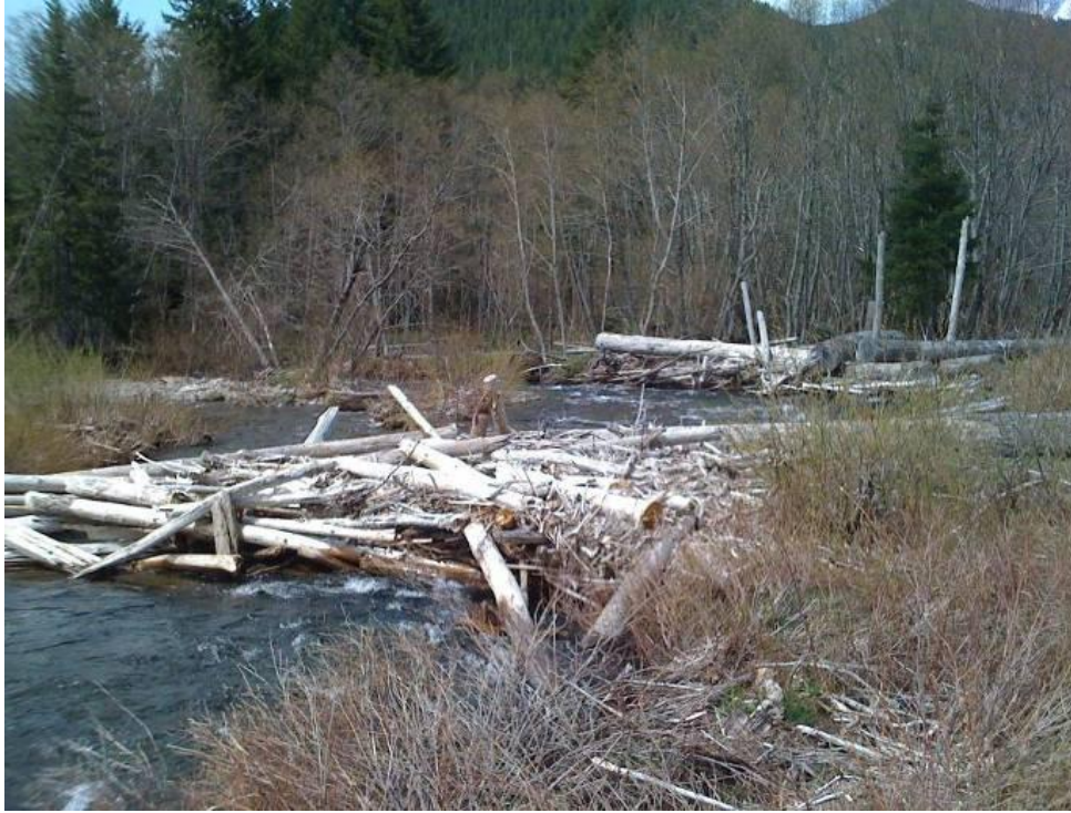
Figure 19. Log jam constructed in 2007. Photo taken 2 years after construction and after a 5-year return interval flood event (West Fork Hood River, OR, Inter-Fluve, Inc.).
