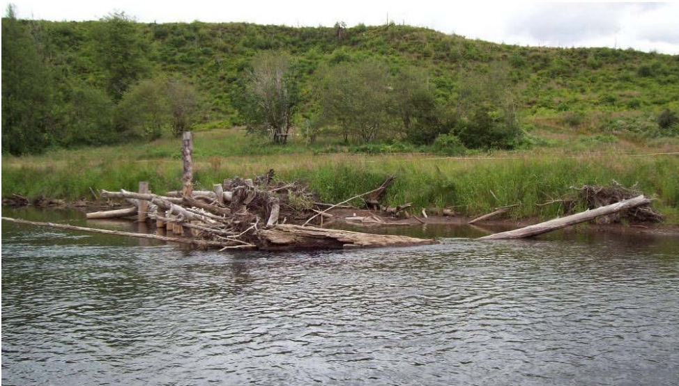
Figure 12. Log pinned to installed piles (Grays River, WA, Lower Columbia Fish Enhancement Group).
