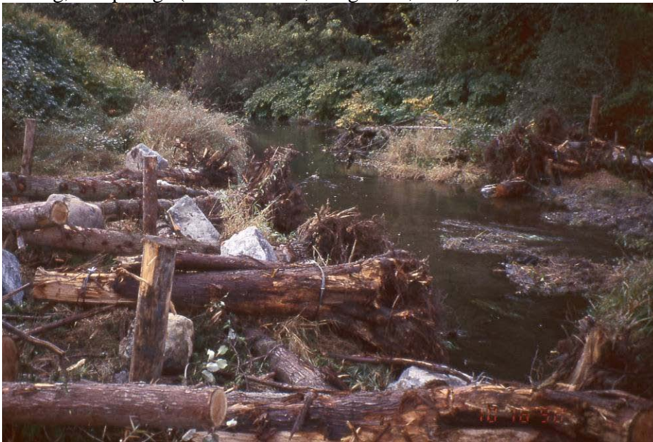
Figure 10. Large wood anchored using a combination of techniques; rock ballast, cabling, and pilings (Samish River, Skagit Co., WA).
