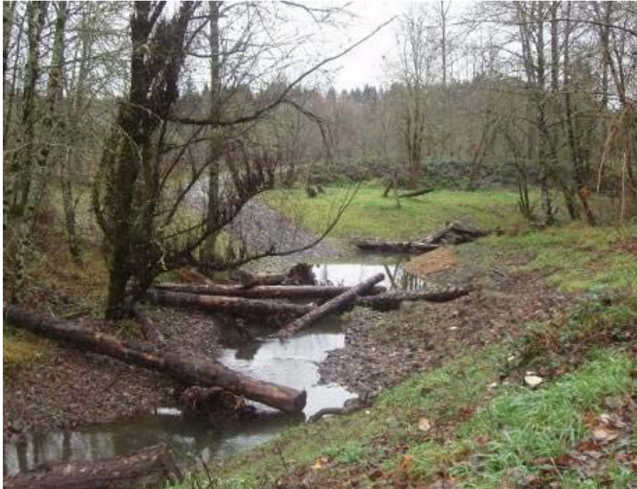
Figure 4. Lower side channel that is a groundwater-fed channel connected to the river only at the downstream end. A constructed infiltration gallery was used to increase the flow to this channel (Inter-Fluve, Inc.).
