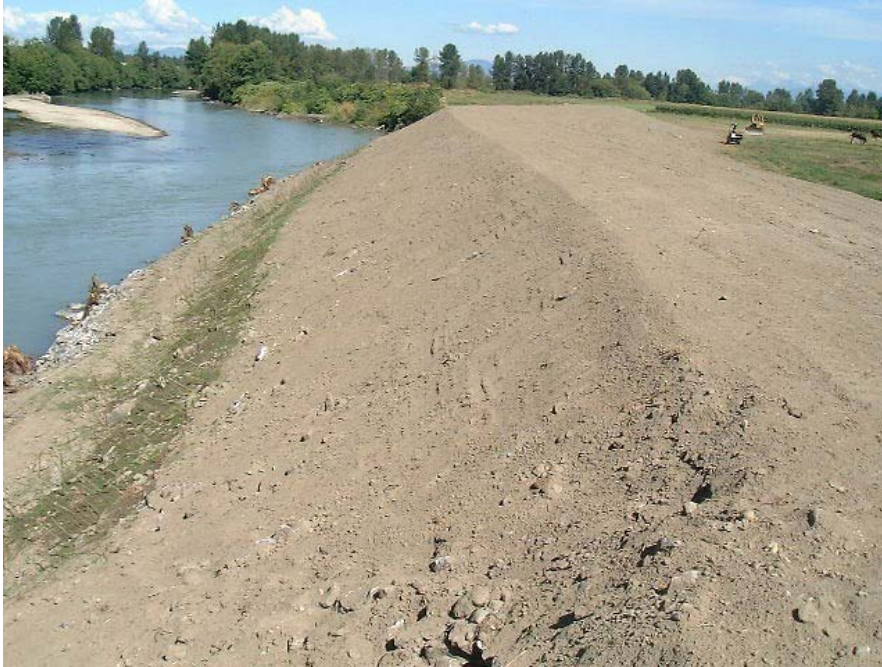
Figure 26. Dikes have been used throughout history to disconnect channels from their floodplains.
