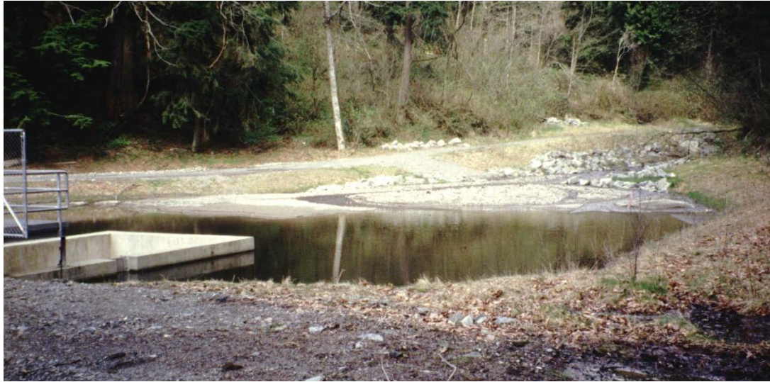
Instream Sediment Detention Basins Figure 6: Maplewood Creek sediment basin, King County. Looking upstream at sediment basin. High flow overflow structure in on right, inlet stream on right. Low flow outlet structure is a fishway off the picture on the left.
