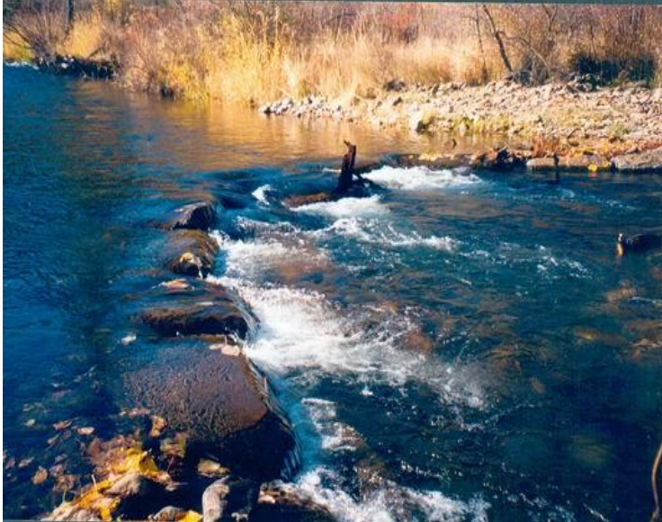
Figure 1. Rock weir. Cedar Creek, WA.
