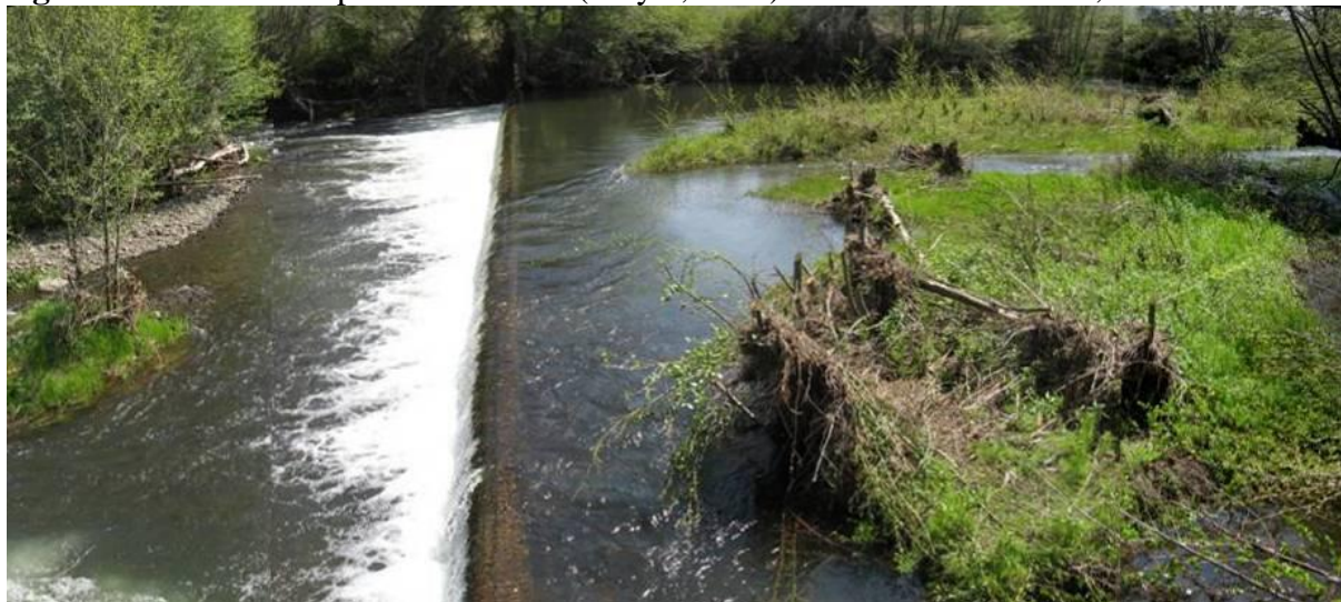
Figure 10. Satus Dam prior to removal (May 8, 2008). Source: Inter-Fluve, Inc.
