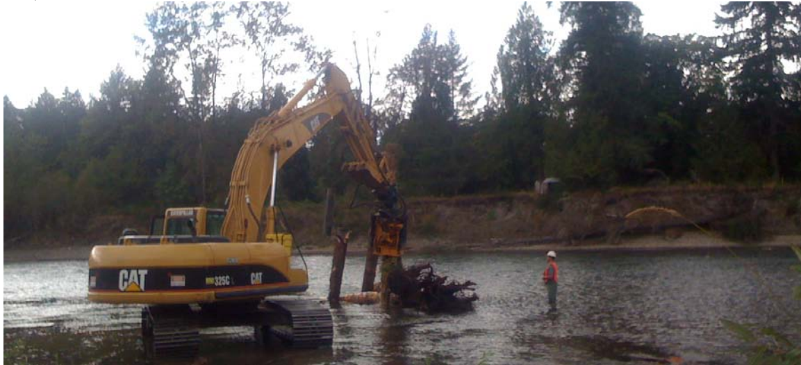
Figure 14. Logs installed with vibratory pile driver (Lewis River, WA, Inter-Fluve, Inc.).
