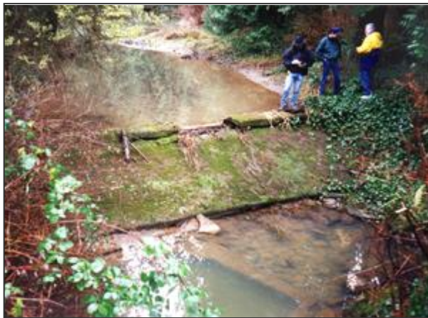
Figure 5. Fish barrier dam (left) replaced by roughened channel / constructed riffle (right). Johnson Creek, OR.
