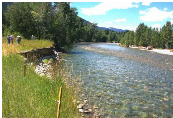
(c) Bank erosion. Source: Paul Bakke
