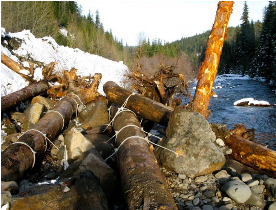
Figure 15 Logs cabled to boulder ballast (Klickitat River, WA, Inter-Fluve, Inc.).
