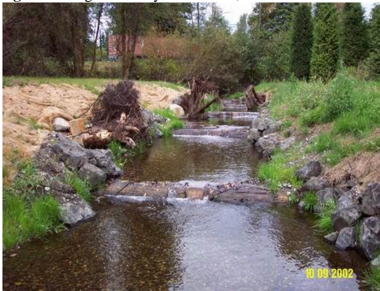
Figure 2. Log weirs. Hylebos Creek, WA.
