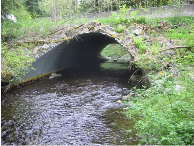
Figure 2.1: No-slope culvert, Johnson Ck, Mosquito Lake Rd.
