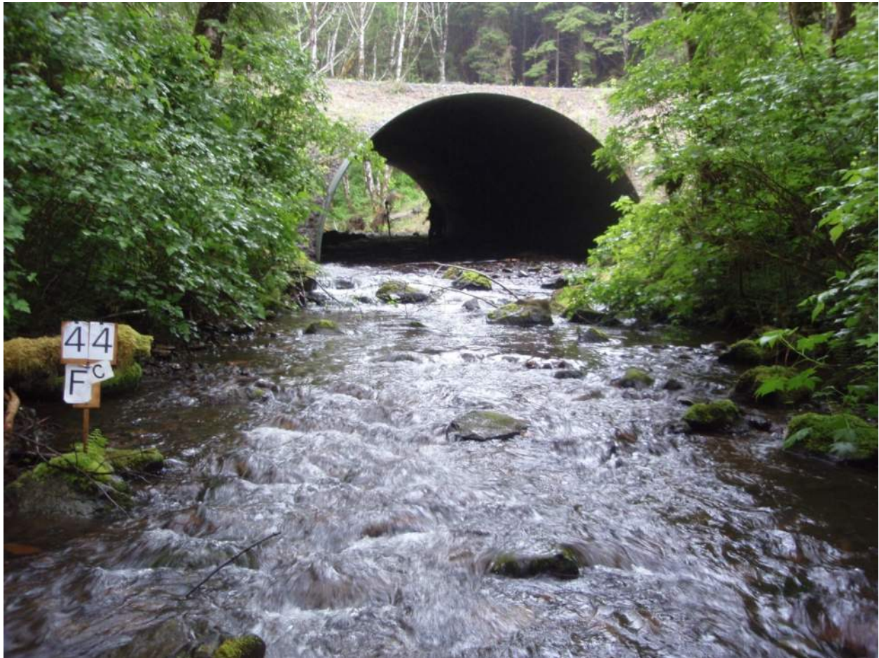
Figure 3.1: Stream simulation culvert, Newberry Ck.
