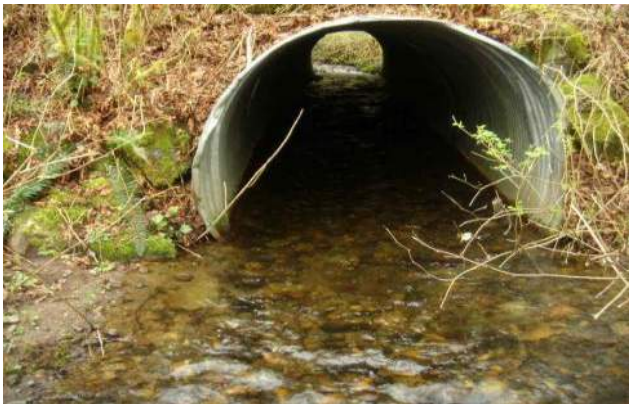
Figure 3: Left photo : No-slope culvert, approx 1996; Duane's Ck, forest road, Snohomish Co.
