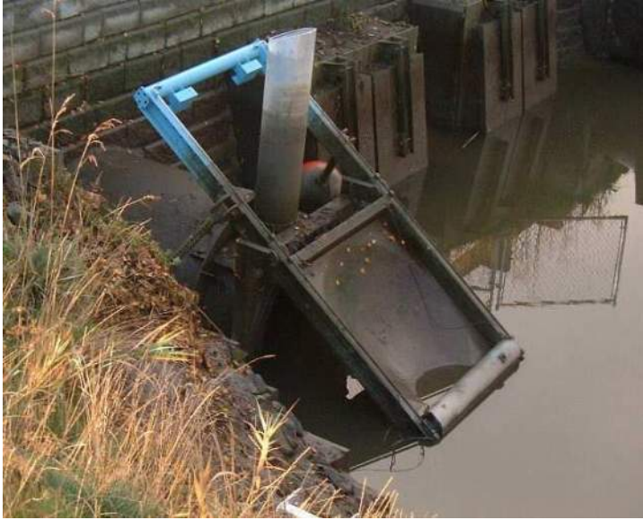
Figure 10.5: Edison Slough self-regulating tide gate.
