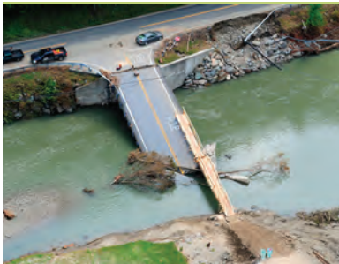
A collapsed bridge in Vermont after Hurricane Irene. Credit: Lars Gange and Mansfield Heliflight
